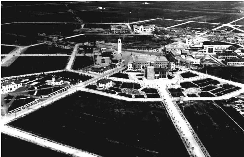
Figure 32: Oriolo Frezzotti/Carlo Savoia, Littoria (today Latina) under construction, 1933.
